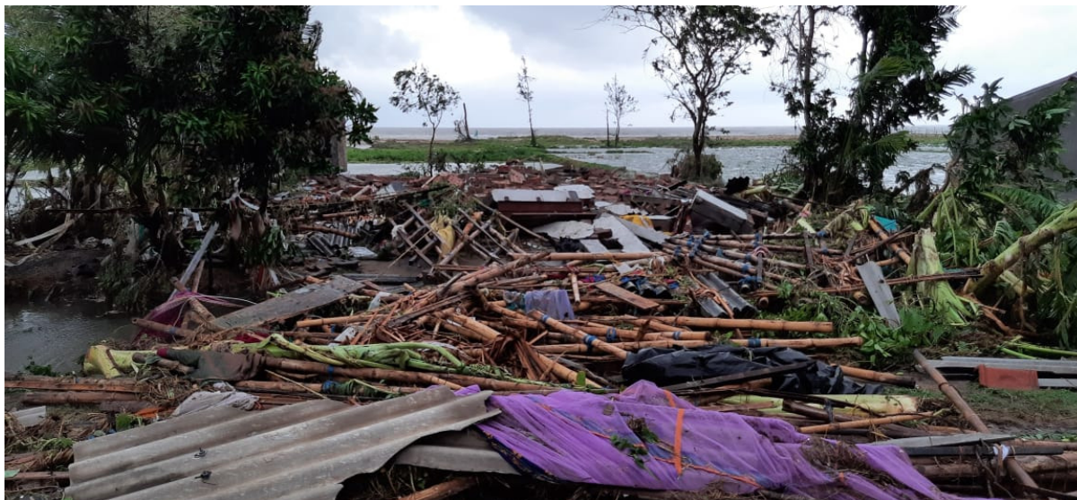
Disaster in Shoula 3 Fish Landing Centre
